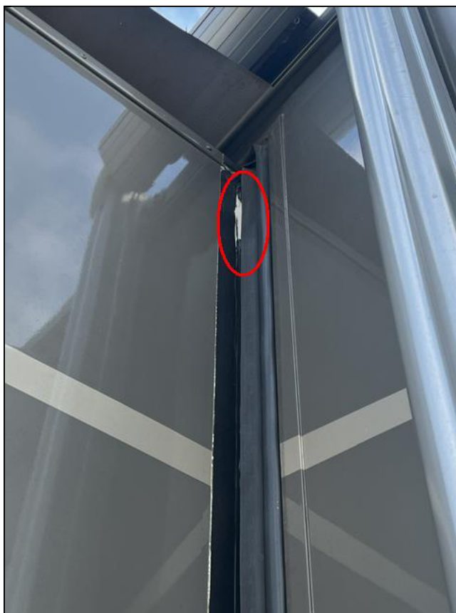
Damaged Tape
