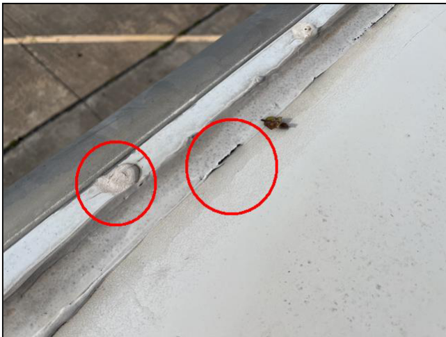
Deteriorating Sealant
