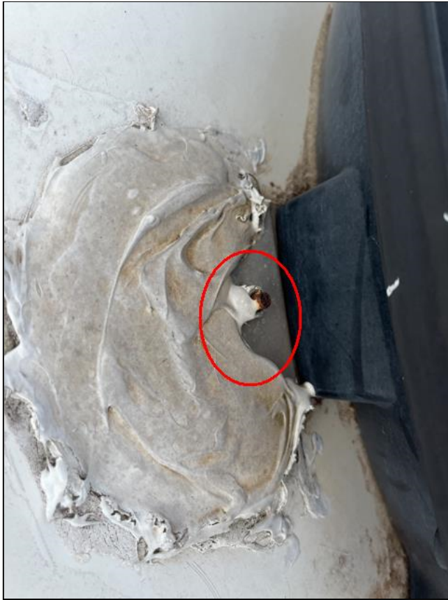
Deteriorating Sealant
