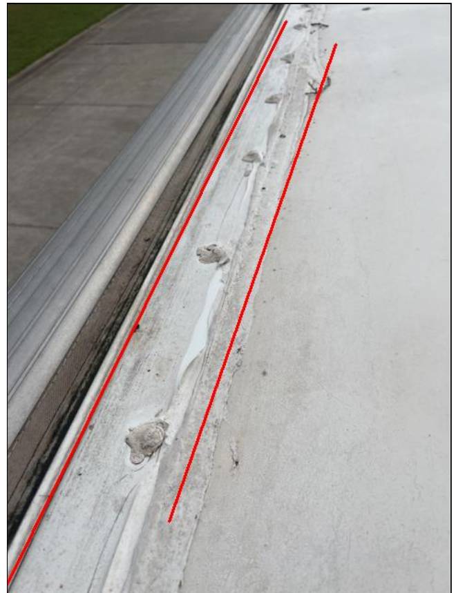
Deteriorating Sealant
