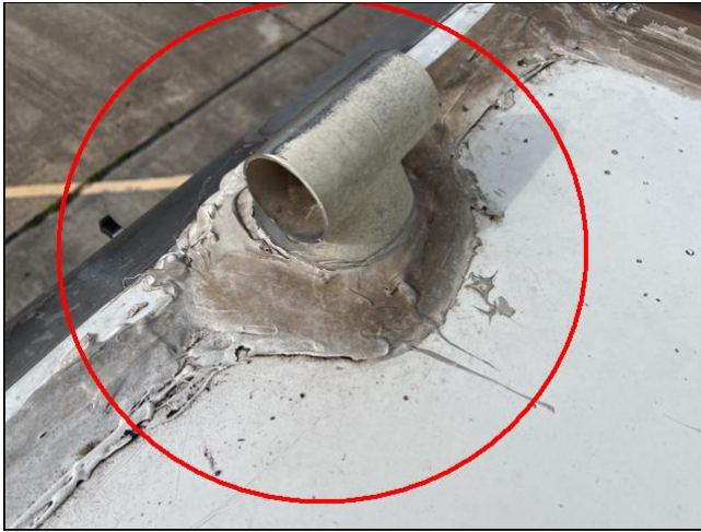
Deteriorating Sealant
