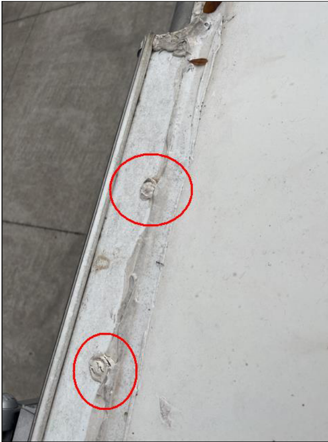
Deteriorating Sealant
