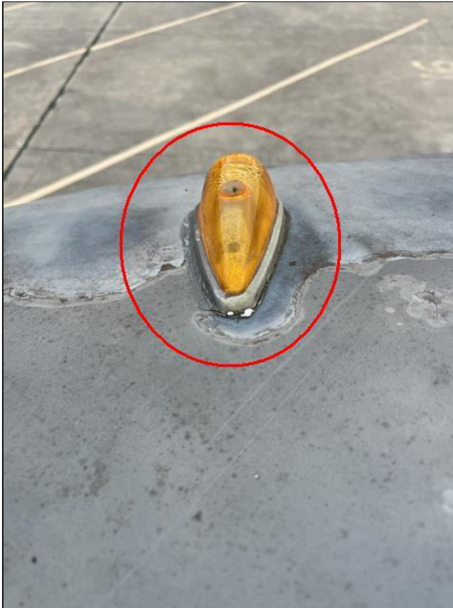
Deteriorating Sealant
