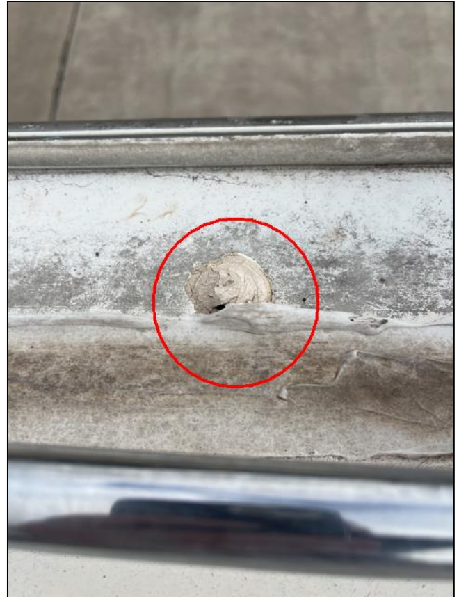
Deteriorating Sealant
