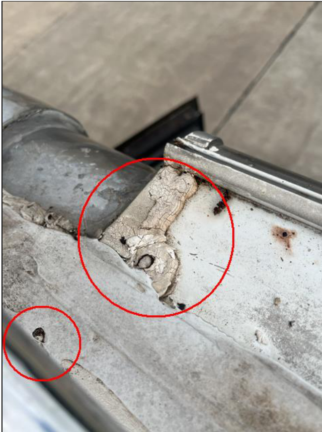
Deteriorating Sealant
