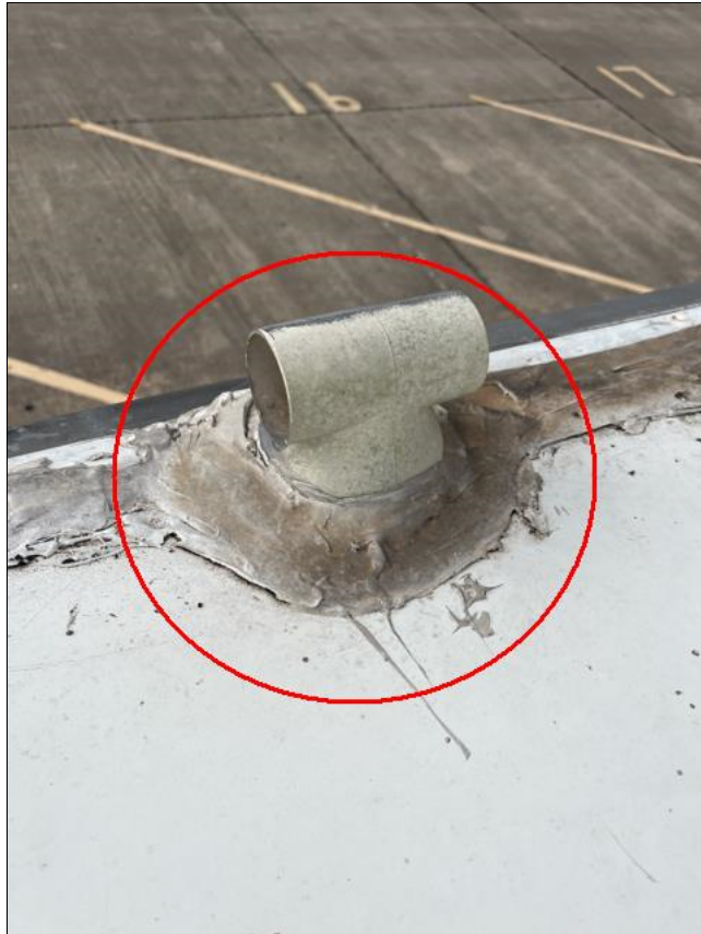
Deteriorating Sealant
