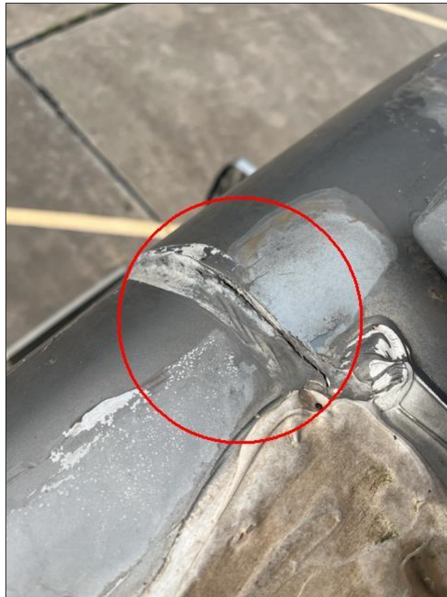
Deteriorating Sealant
