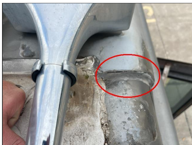
Deteriorating Sealant
