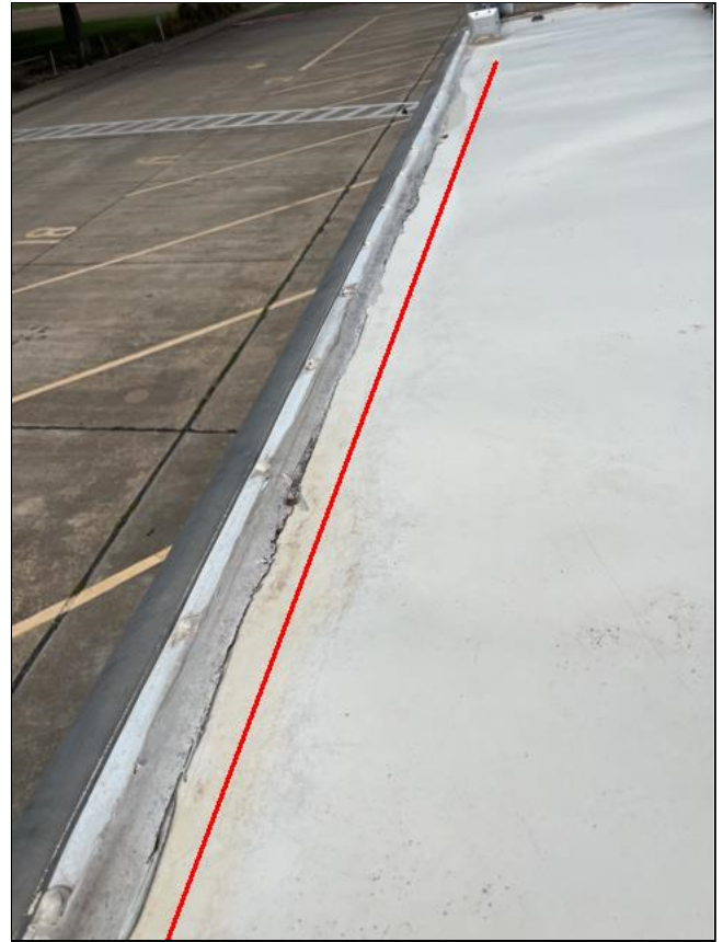
Deteriorating Sealant
