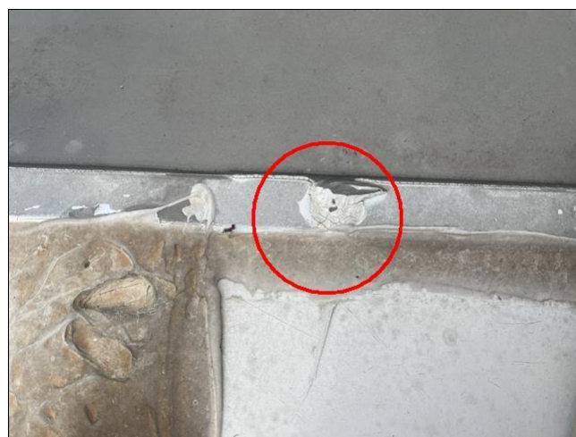
Deteriorating Sealant
