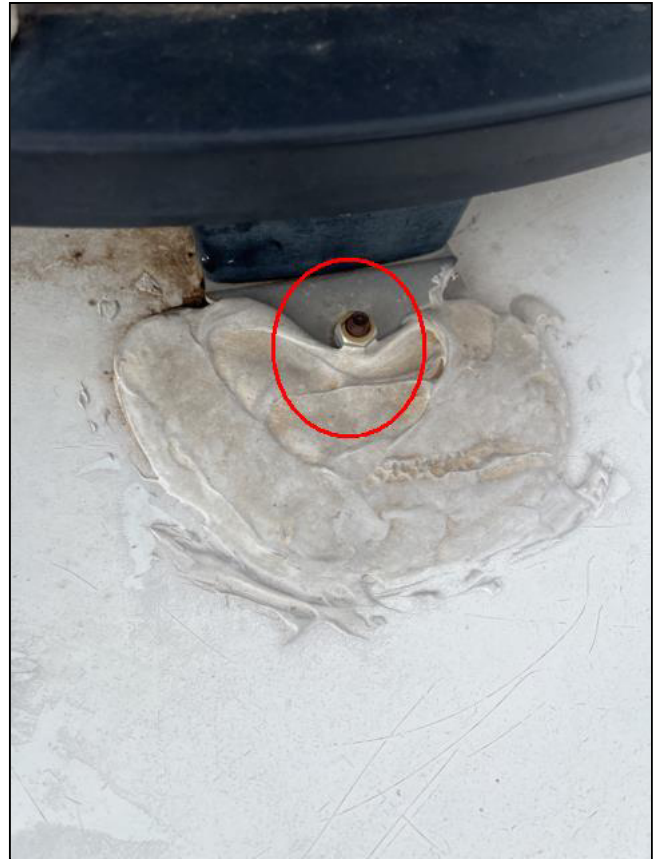
Deteriorating Sealant
