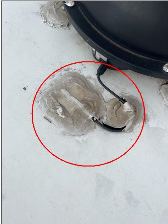
Deteriorating Sealant
