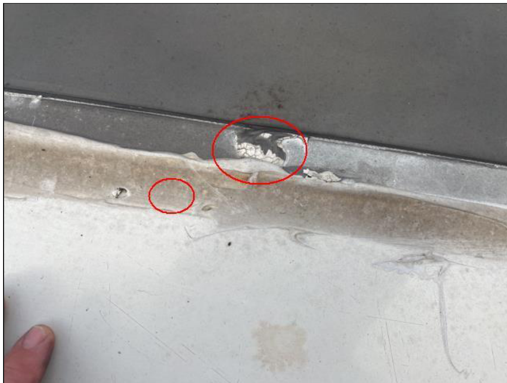
Deteriorating Sealant
