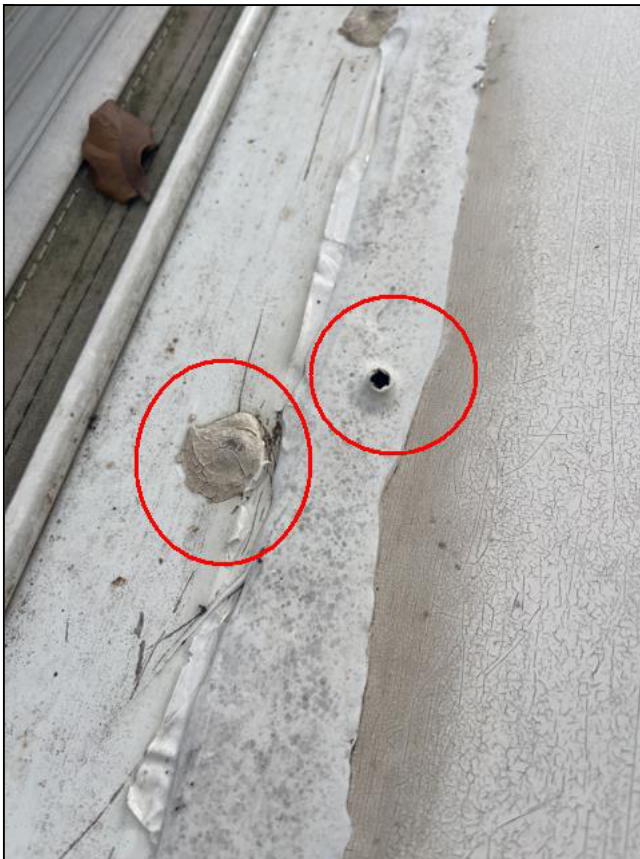
Deteriorating Sealant
