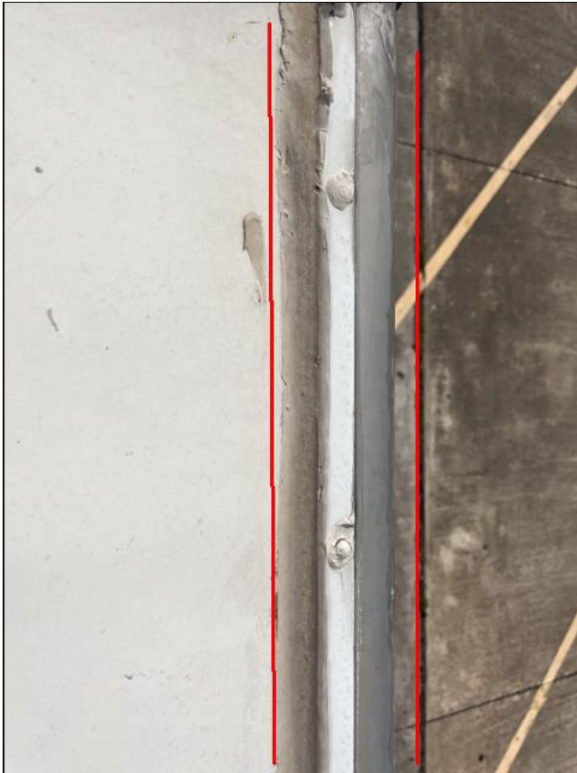
Deteriorating Sealant
