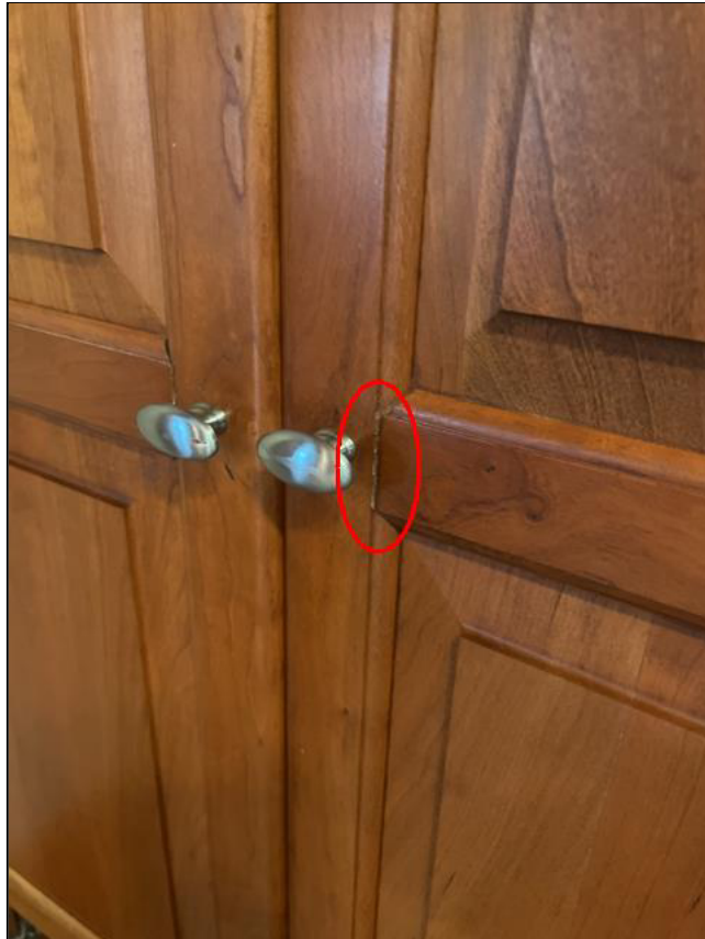
Damage to Cabinet
