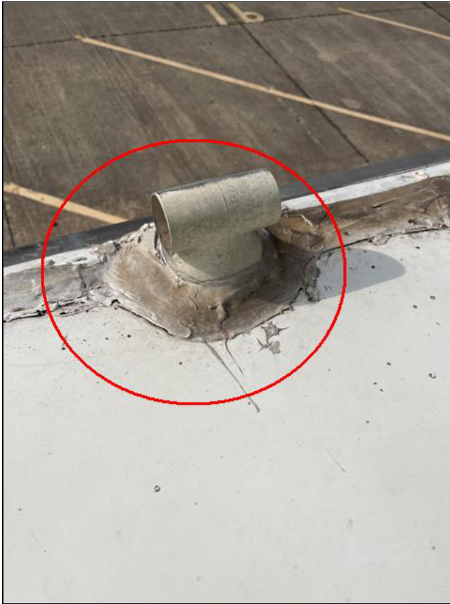
Deteriorating Sealant
