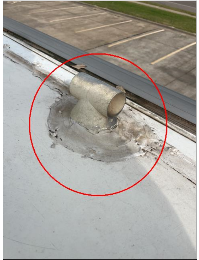
Deteriorating Sealant
