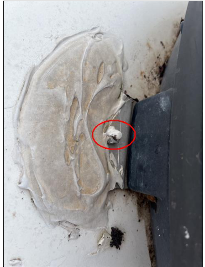
Deteriorating Sealant
