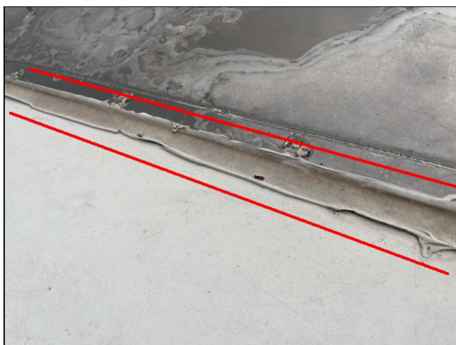
Deteriorating Sealant
