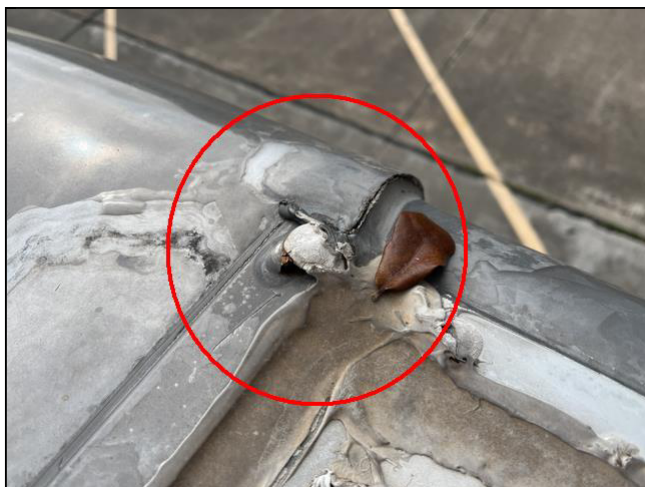
Deteriorating Sealant
