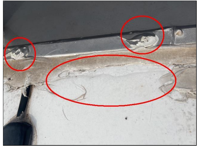
Deteriorating Sealant
