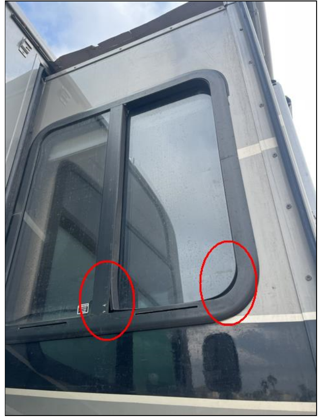
Decaying window seals
