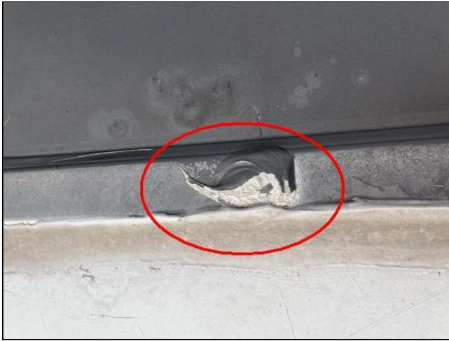
Deteriorating Sealant
