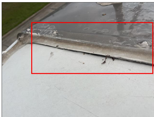
Deteriorating Sealant
