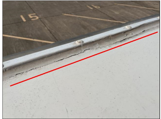
Deteriorating Sealant
