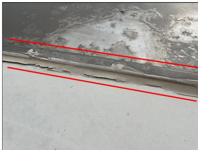
Deteriorating Sealant
